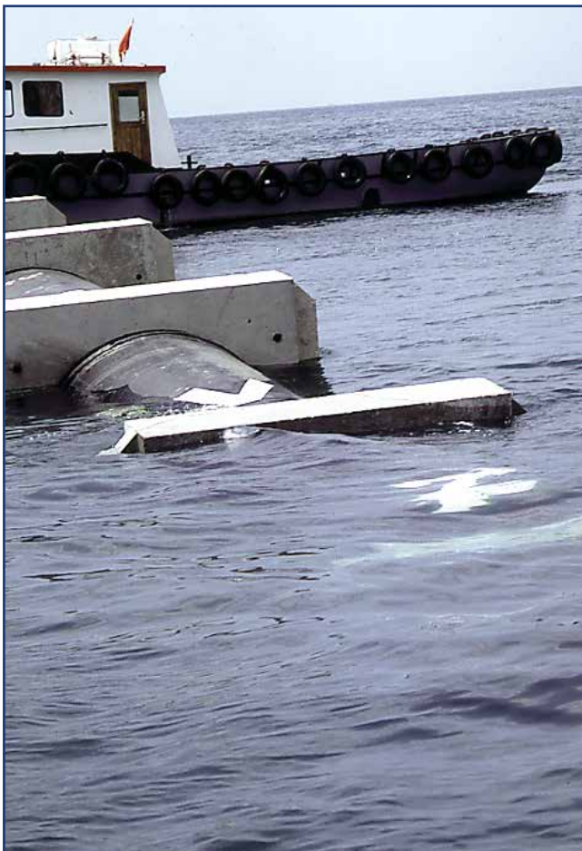
Picture 1.1.10 - Pictures showing bending ability of Dizayn pipes of 1600 mm dia. PN 4 produced for sea discharge project in Buyukcemkece / Istanbul.
