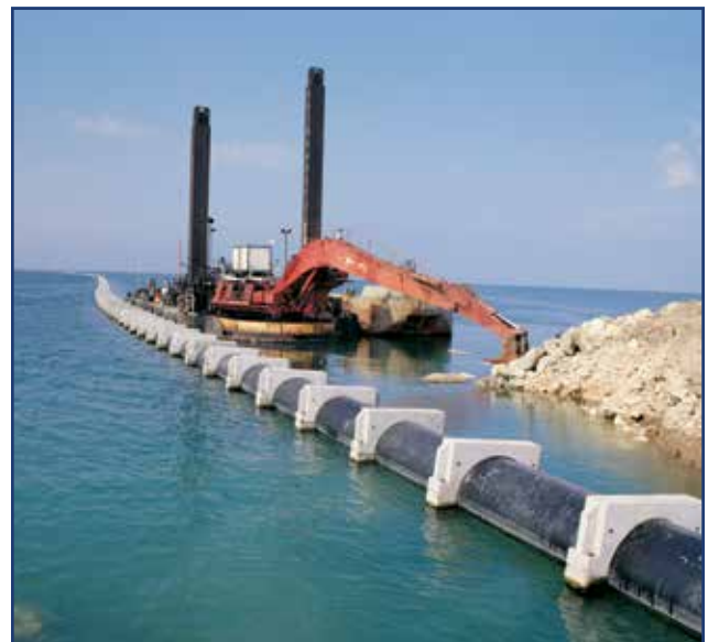
Picture 1.1.2b - Pipes another view from sea discharge application of 1600 mm o.d.
