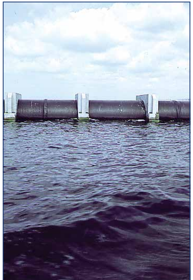
Picture 1.1.10 - Pictures showing bending ability of Dizayn pipes of 1600 mm dia. PN 4 produced for sea discharge project in Buyukcemkece / Istanbul.
